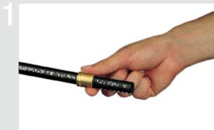
Slide the compression sleeve over the pipe
